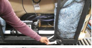
Pictured to the right is the inside of the spa behind the front door. The electrician now has access to connect the spa for power. While the front door is off, refer to page 10 for instructions on ensuring the plumbing fittings are secure (but do not be tempted to over-torque or over-tighten these fittings).
