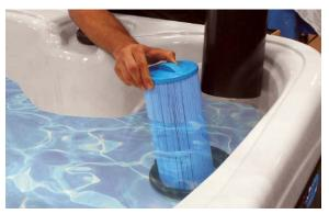
Unscrew the cartridge and remove it.
